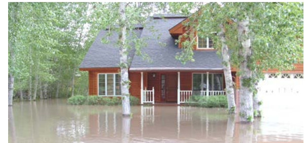
May 2006 Flooding in Hailey
