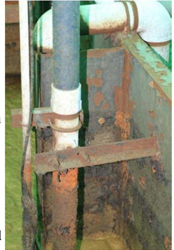
*Shown here, many parts of the 1974 facility are corroded and rusting, causing safety concerns.*
